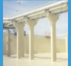
Waste Water Treatment
