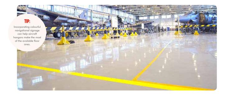
Aggregates can be broadcast into resin floor coatings to enhance the floor's anti-slip profile while maintaining an attractive, seamless coating. The aggregate size can be customised to match the specific requirements of individual sites. Broadcasting aggregates into a resin floor also has the added benefit of increasing its durability and lengthening its longevity by creating a much tighter matrix.
