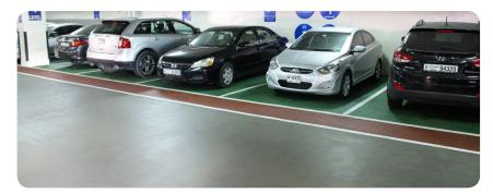
► In 1999, 32,000m<sup>2</sup> of the solvent free polyurethane car park deck coating system Deckshield ID was applied within the Deira City Centre's parking facility – and it is still in use today five years after its guarantee expired!
