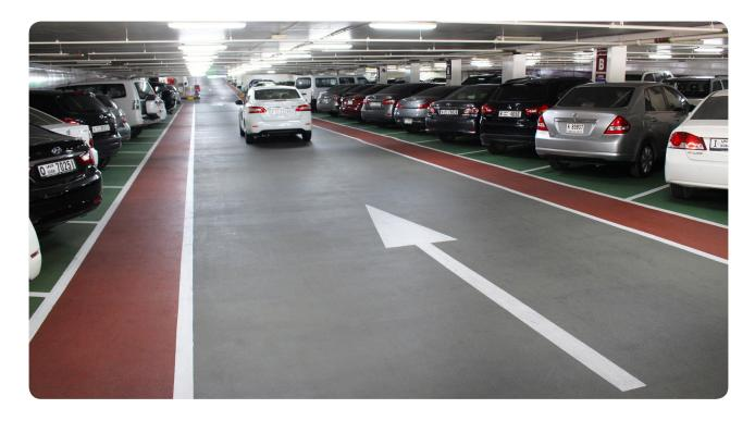
epoxy primer. The epoxy primer in hybrid systems is rigid and therefore makes it more prone to failure than the polyurethane primer of Deckshield, meaning that Deckshield is better able to withstand deflection within the slabs or decks of car parks caused by intense multiflow traffic.
